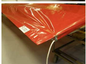
Drill holes in the tarpoulin and mount the rope clamps on both sides of the gable. Cut the tarpoulin accordingly to the pictures.
