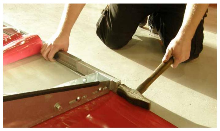
When pushing the pipes into the gable, it is good to have a hammer to knock in the last bit.
