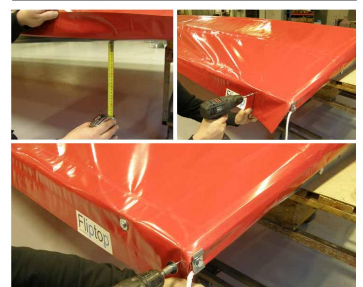
Screw the tarpoulin along with the long sides with montage screws (5,5x20 + washer) that came with the tarpoulin.
