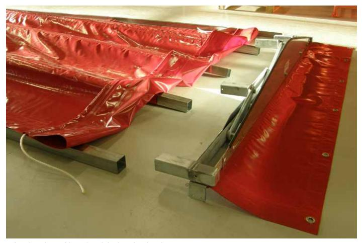
Bring the other gable and push in the tubes into it. if you must have a flap on the end should be installed before this step.
