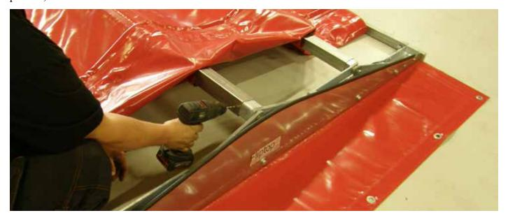
Each tube (the three inner 60x60x2) must now be drilled like the picture, and stuck together with M10x75 (1p), 11x28x2 (2p) M10 lock nut (1p) per tube.
